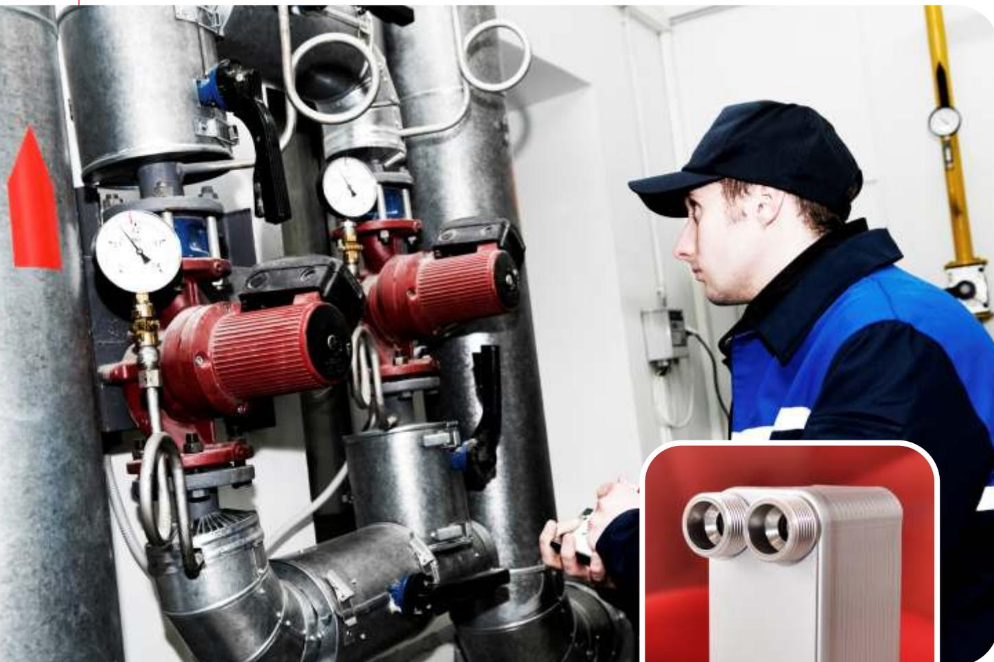
A brazed plate heat exchanger (BPHE) is normally self-cleaning, thanks to highly turbulent flows. In applications with a high risk of fouling or scaling, e.g. due to high temperatures, hard water, or high pH levels, cleaning may be required to maintain efficiency. This is achieved quickly and easily with Cleaning in Place, a method of cleaning the interior surfaces of closed systems by circulating a fluid. Disassembly is not required.
