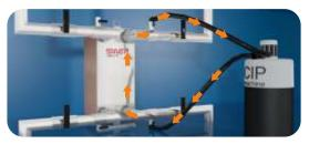
Connect the CIP machine via inlet/outlets on front or back. Pump the solution into the BPHE using the lower connection to expel air. Reverse the flow direction every 30 minutes.
